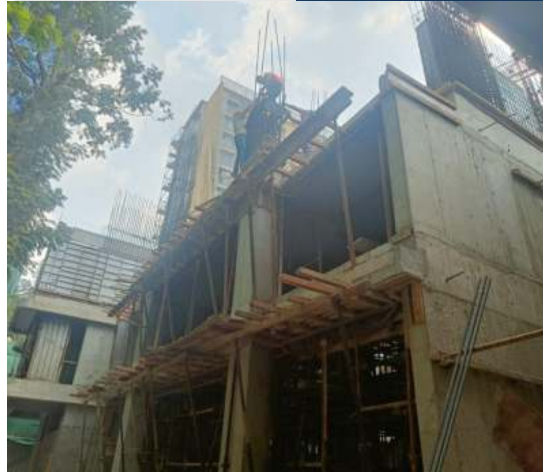
2nd Floor Slab Casted
