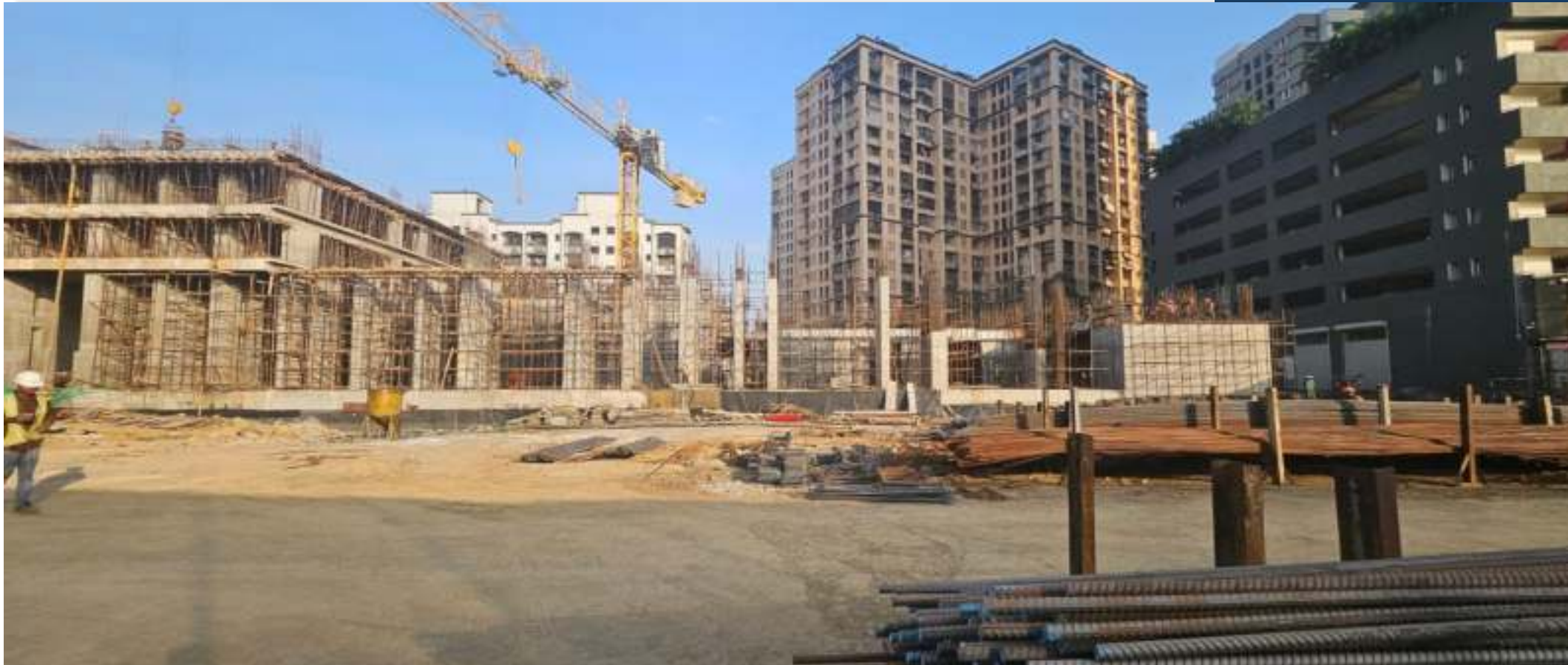
Tower B – Podium WIP
