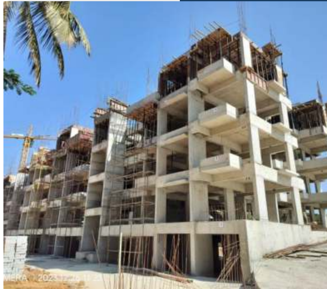
Tower CD - West View
