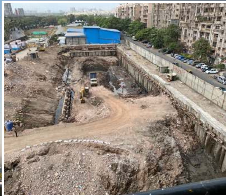
Piling Work Completed
