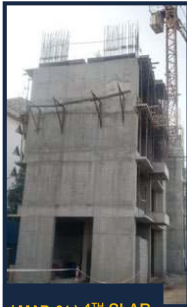
( MAR-21 ) 4 TH SLAB
